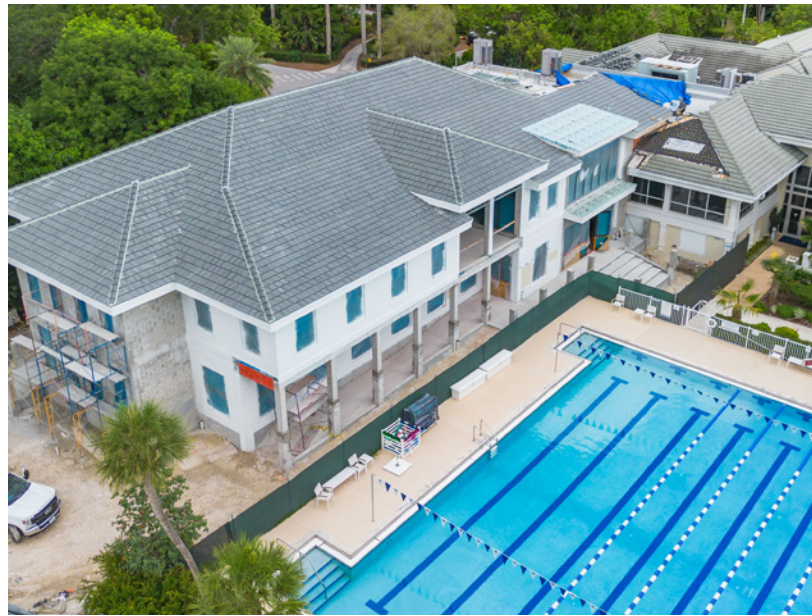
Spa renovation and expansion, May 18, 2026.
