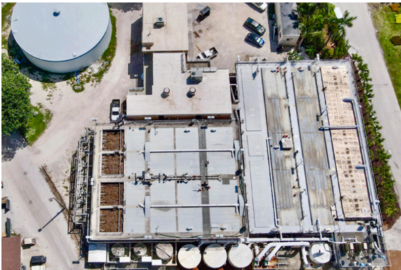
NKLUC's Advanced Wastewater Treatment Plant (Photo by Jorge Arteaga).
