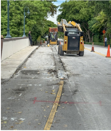
Yellow curbs on Ocean Reef Drive Bridge are removed and electrical lines were relocated.
