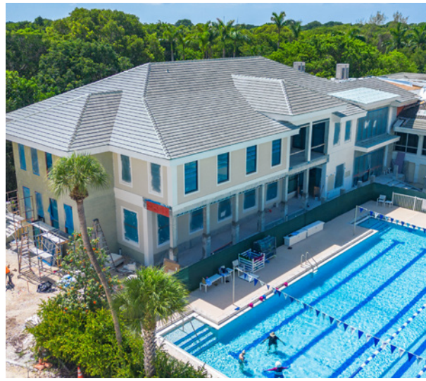
Spa renovation and expansion, June 22, 2026.
