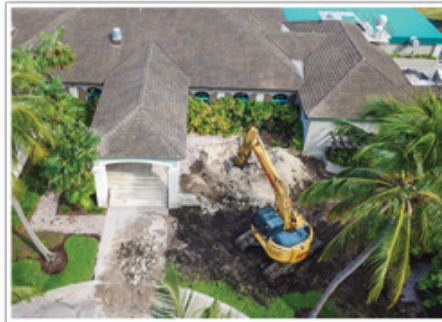
Demolition Progress: July 16, 2020
