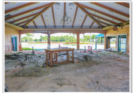
Demolition Progress: July 21, 2020
