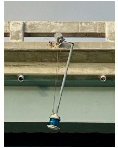
These pictures show three safety hazards – a damaged Navigation Aid, one without a number, and a damaged bridge light. If you see something like this, please take a picture and share it with someone from the Coast Guard Auxiliary.
