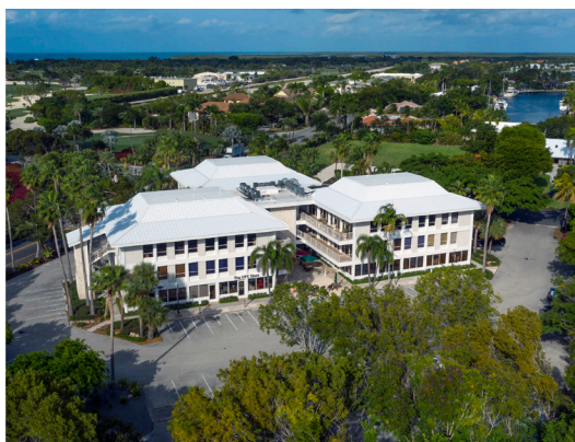
Plaza Building | Commercial
