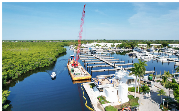
Construction has officially begun on the Marina seawall enhancement project, which will replace 1,100 feet of seawall from the Marina Fuel Dock to H Dock.
