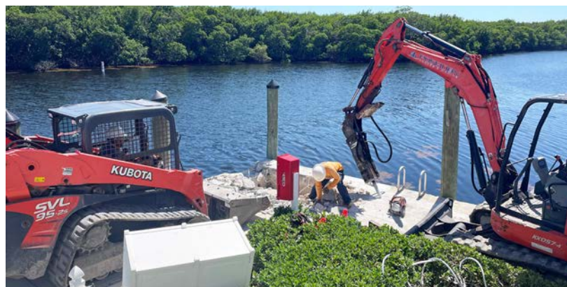
Progress on the Marina seawall enhancement project, photographed May 1, 2023
