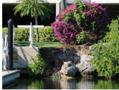
Proof that waves erode the coral walls, causing boulders to fall into the cove.
