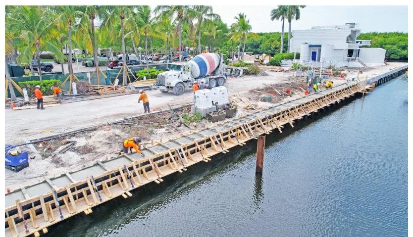
Concrete cap pour near D Dock, photographed June 16.
