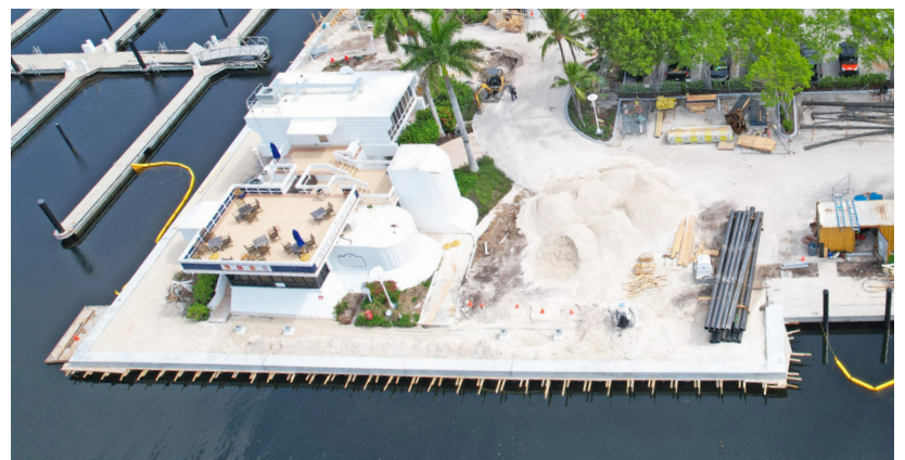
Fuel Dock and D Dock progress seven days later on June 16.
