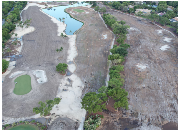
Dolphin Hole #6 progress, photographed May 26.
