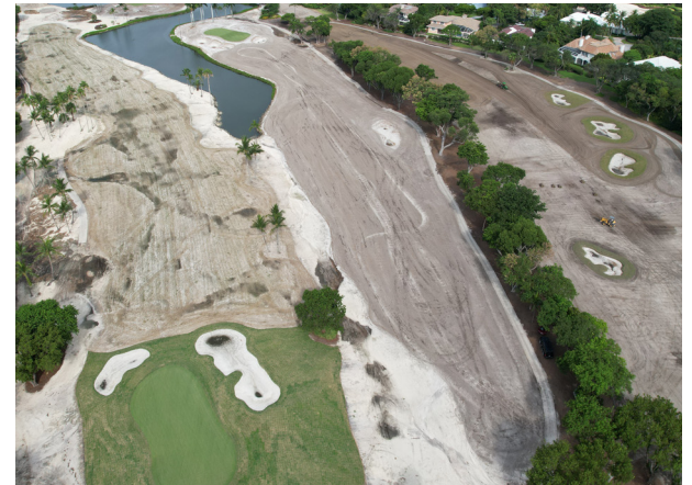
Dolphin Hole #6 progress, photographed June 22.
