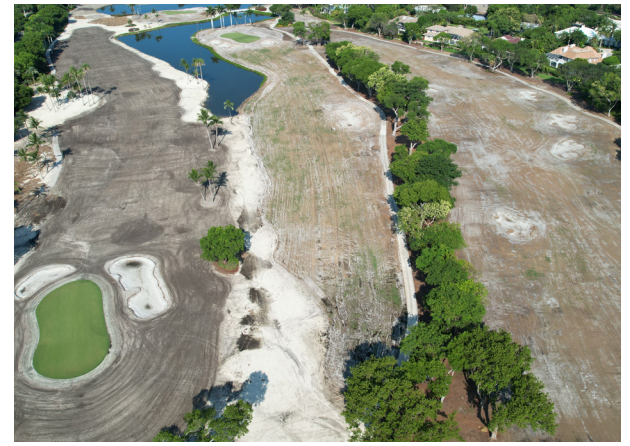
Dolphin Hole #6 progress, photographed June 2.
