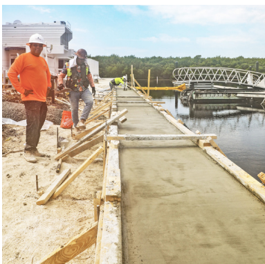
Concrete cap pour near D Dock, photographed June 16.
