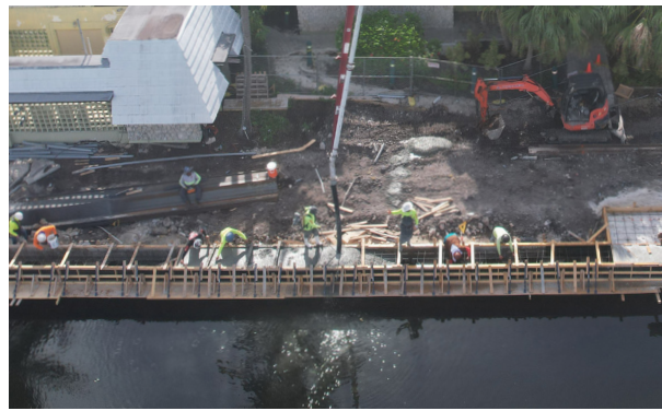
The seawall in front of Marina Fitness Center, pictured left on July 14, underwent concrete pour this week on July 24 (pictured right).
