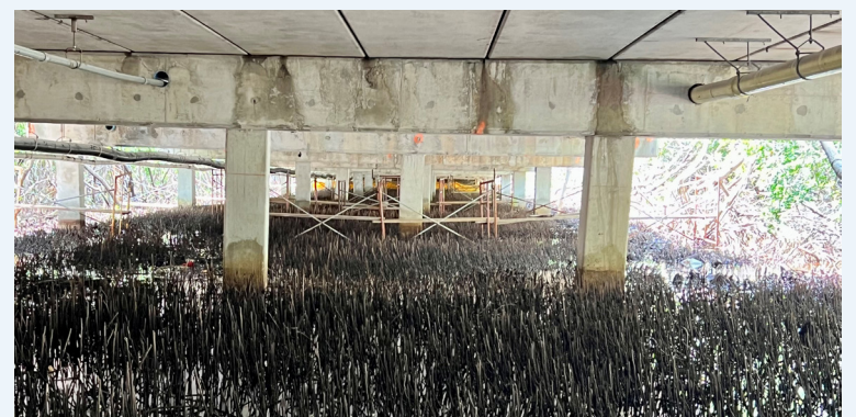
Bridge crews work on essential repairs beneath South Harbor Bridge.
