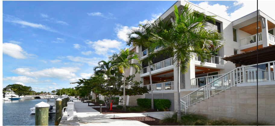
121 Marina 105 4 BD/4.5 BA | 3,364 a/c sq. ft. | 1st Floor | Extra Lanai Space Stairwell to Dock | $10,250,000 furnished | 2541
