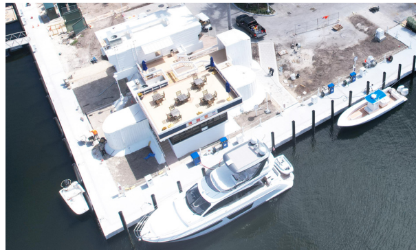
Fuel Dock as of July 7
