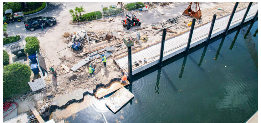
H Dock construction photographed August 17, 2023.
