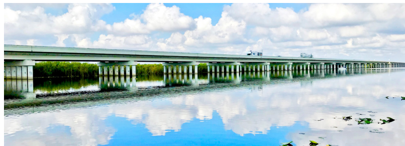
Everglades Foundation Tamiami Trail bridges
