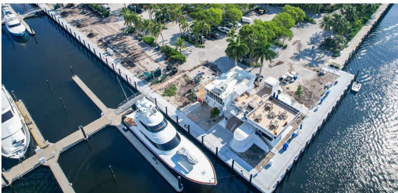
View of the reinstated Fuel and D Docks as of August 25, 2023.
