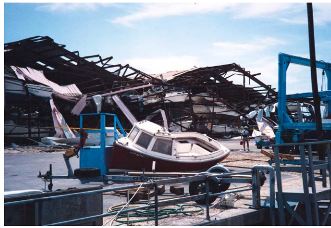
The Boat Barn after Hurricane Andrew on August 25, 1992 .
