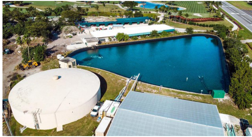
Reverse Osmosis irrigation plant
