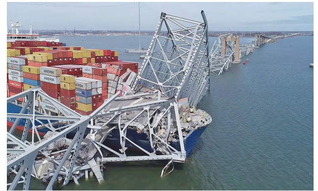
Allision of the container ship, Dali, with Baltimore's Key Bridge—March 26, 2024. Photo: NTSB.
